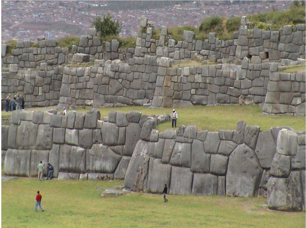
6 Sacsayhuaman is famous for three walls from giant stones, erected one above the other; the dimensions of the blocks diminish with the height.
